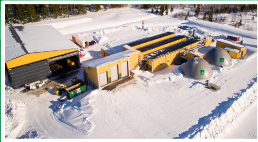
BioGTS® Biogas plant, Haminan Energia Ltd., Virolahti, Finland
