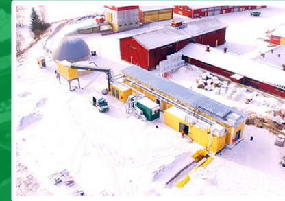
BioGTS® Biogas plant, Suupohja Vocational School, Kauhajoki, Finland
