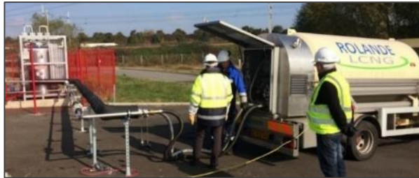
Bio-LNG transfer to the mobile transport station
