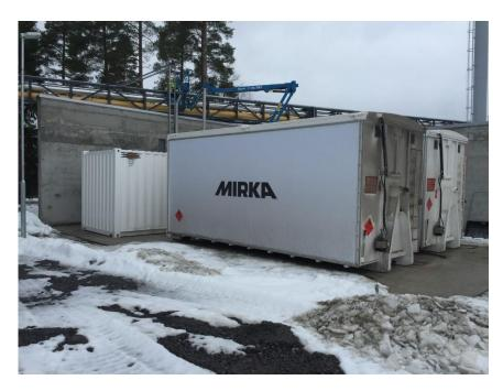
Bio methane containers, gas pressure 250 bar and pressure reduction station, built by Adven.
